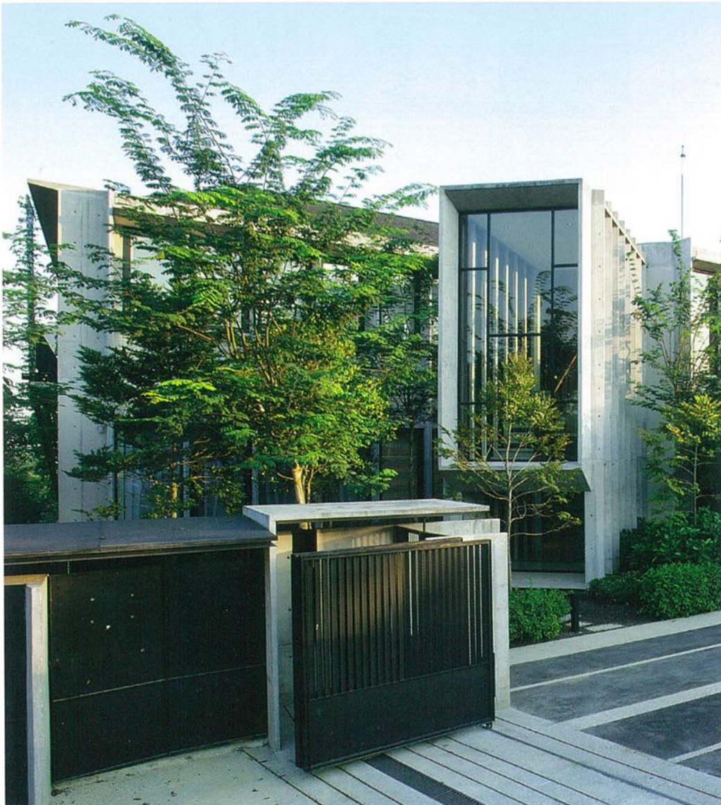
The facade, showing the stairwell with its tall windows that open up to the views.
